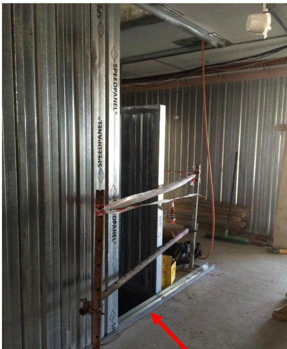
The casualty was standing on a bucket at the edge of the air duct applying sealant to the joins between the panels. There was no fall prevention system in place at the time of the incident. **This attempt at barricading was installed post incident**
